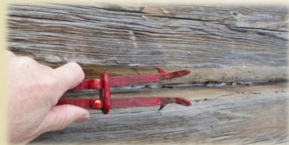
Using the Vara for scribing the logs to fit.
